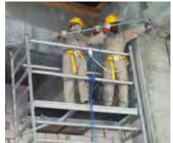
SBT team members installing conduits in parcel area nine.
