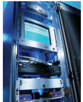
Our Mobility colleagues are currently involved in the modernisation of the Orex line with the installation of the SIMIS S electronic interlocking system above.
